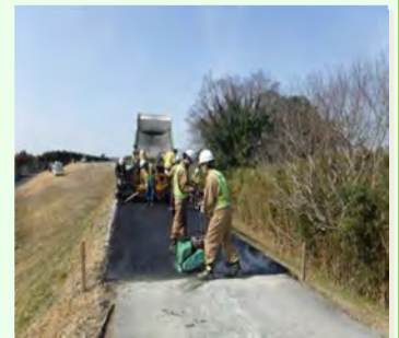
堤防天端の補修状況
