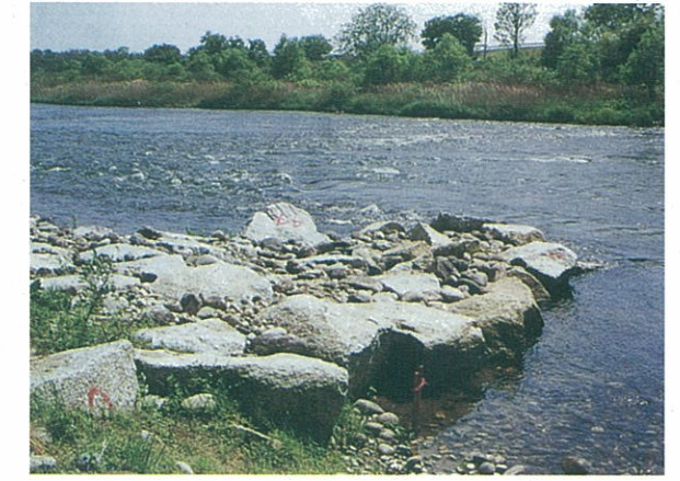
水制工 Spur Dikes on the Yahagi River
