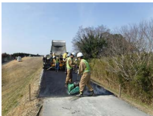
堤防天端の補修状況
