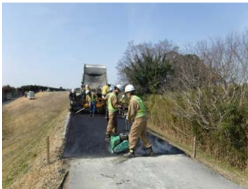
堤防天端の補修状況
