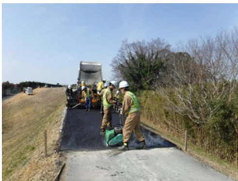
堤防天端の補修状況
