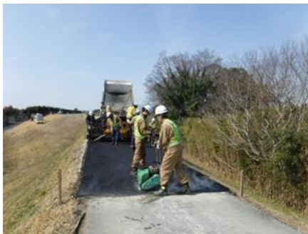
堤防天端の補修状況
