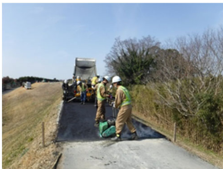
堤防天端の補修状況
