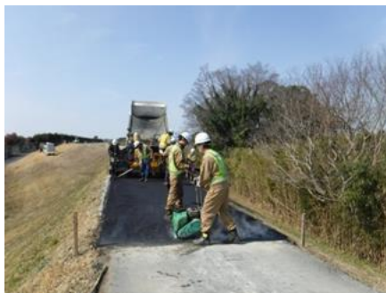
堤防天端の補修状況
