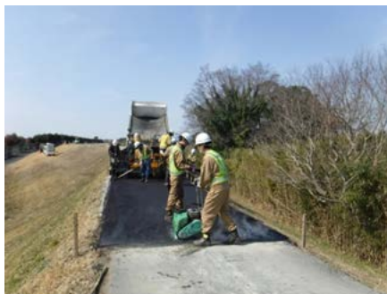
堤防天端の補修状況
