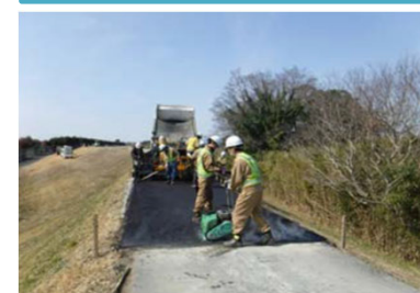
堤防天端の補修状況
