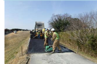
堤防天端の補修状況
