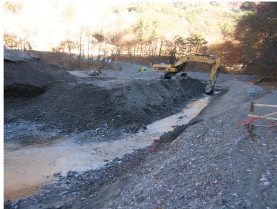
Picture 3 Sediment exclusion work on sand pocket
