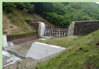
矢立木砂防堰堤
