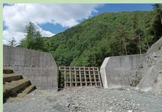
持社沢砂防堰堤
