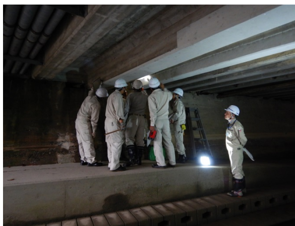
桁の状態を打音点検
