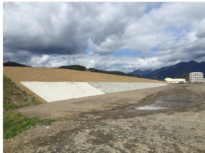
H31安倍川安倍口築堤護岸工事 (10.50k右岸付近)
