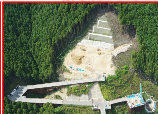
③松戸地区橋梁下部工
