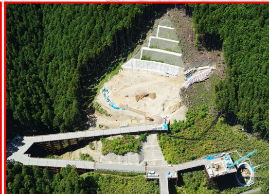
③松戸地区橋梁下部工
