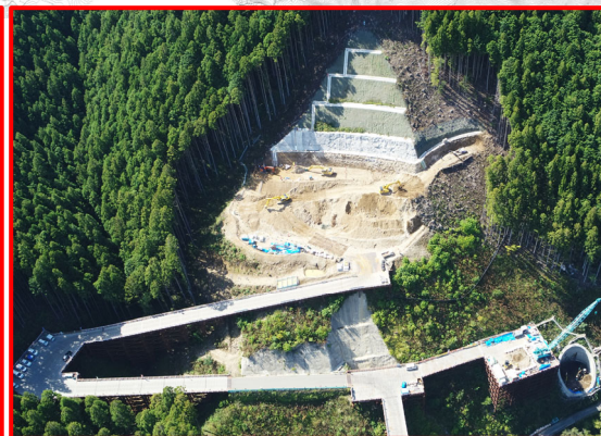
③松戸地区橋梁下部工
