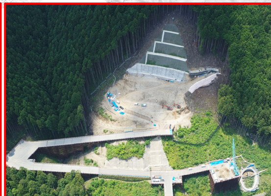
③松戸地区橋梁下部工
