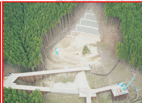
③松戸地区橋梁下部工
