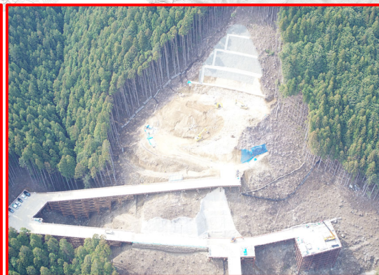
③松戸地区橋梁下部工
