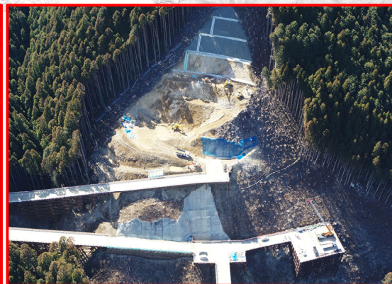
③松戸地区橋梁下部工
