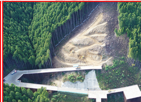
③松戸地区橋梁下部工
