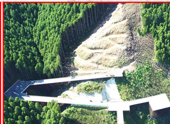
③松戸地区橋梁下部工
