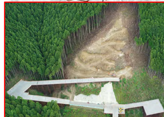
③松戸地区橋梁下部工
