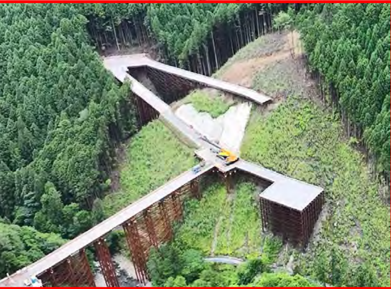
③松戸地区橋梁下部工
