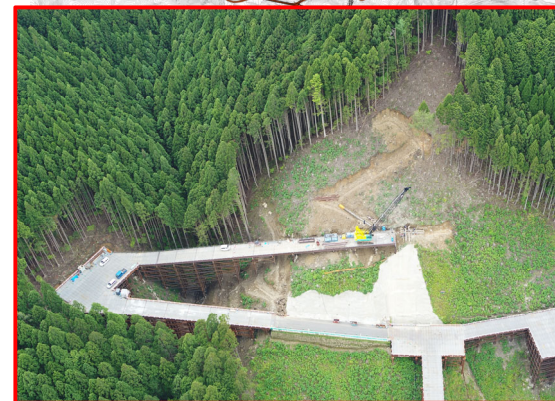
③松戸地区橋梁下部工
