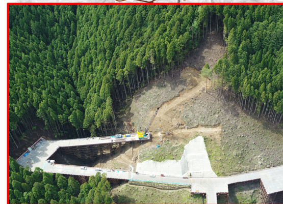
③松戸地区橋梁下部工
