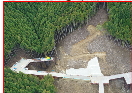
③松戸地区橋梁下部工
