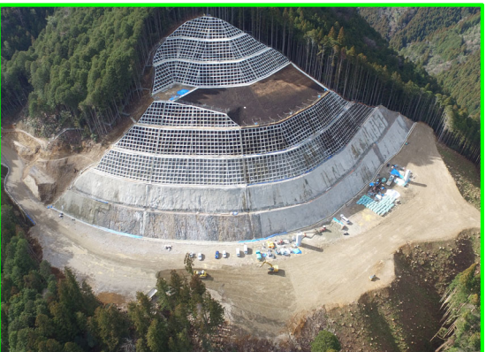
①左岸頂部掘削
