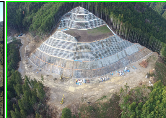
①左岸頂部掘削
