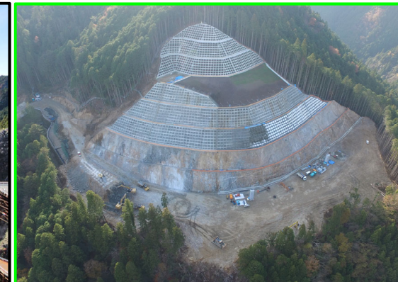
①左岸頂部掘削
