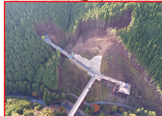
③松戸地区橋梁下部工
