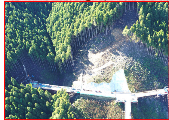
③松戸地区橋梁下部工
