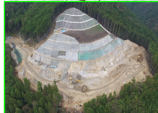
②左岸頂部掘削
