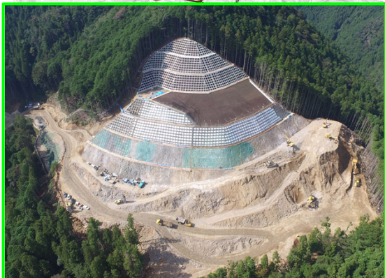
②左岸頂部掘削
