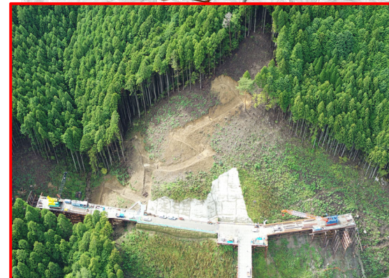
③松戸地区橋梁下部工
