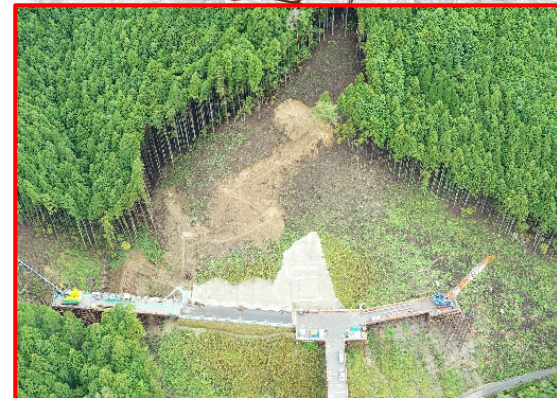
③松戸地区橋梁下部工
