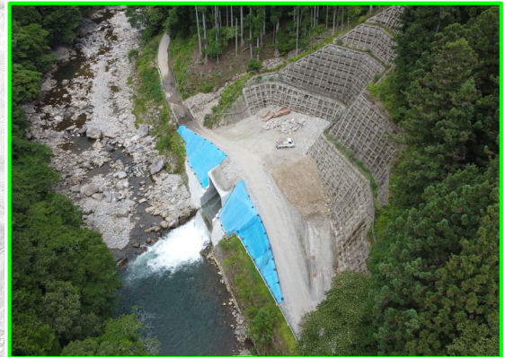
①堤外仮排水路 (吐口側)
