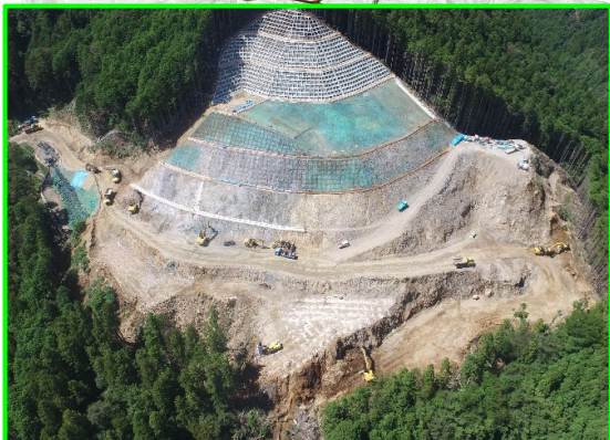
②左岸頂部掘削
