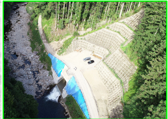
①堤外仮排水路 (吐口側)
