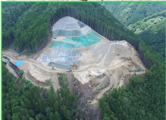
②左岸頂部掘削
