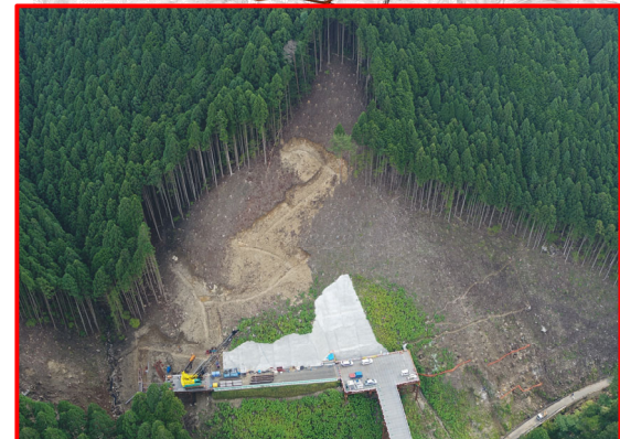
③松戸地区橋梁下部工
