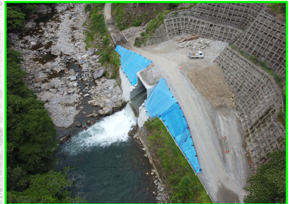
① 堤外仮排水路 (吐口側)
