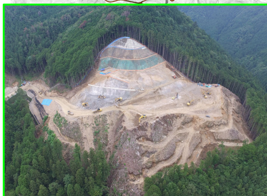
②左岸頂部掘削
