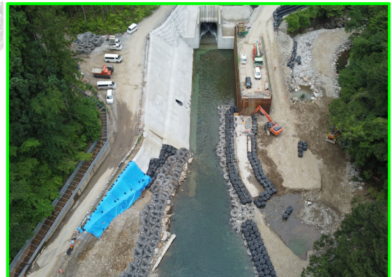
① 堤外仮排水路 (呑口側)
