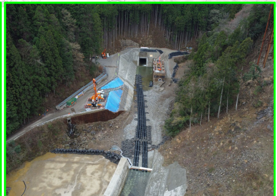
① 堤外仮排水路 (呑口側)
