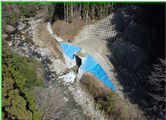
① 堤外仮排水路 (吐口側)
