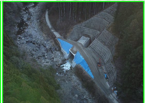
① 堤外仮排水路 (吐口側)
