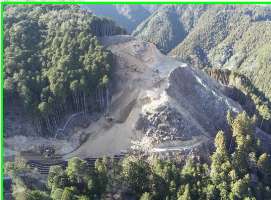
②左岸頂部掘削
