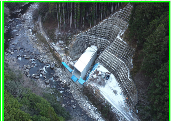
①堤外仮排水路 (吐口側)
