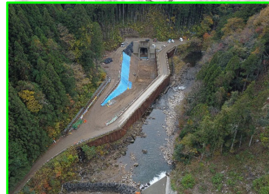
① 堤外仮排水路 (呑口側)
