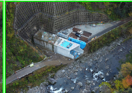
① 堤外仮排水路 (吐口側)
