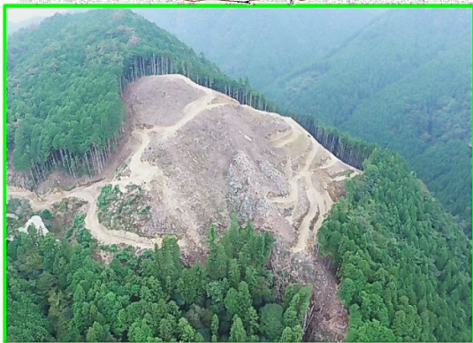
②左岸頂部掘削
