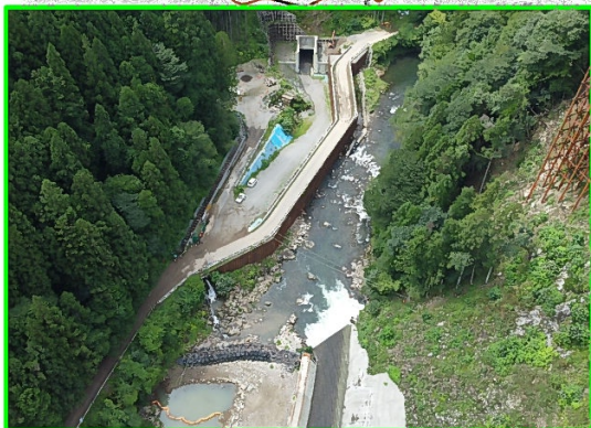
①堤外仮排水路(呑口側)
