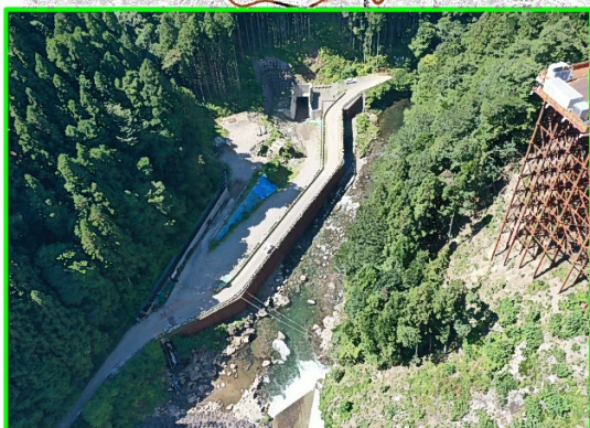
①堤外仮排水路(呑口側)
