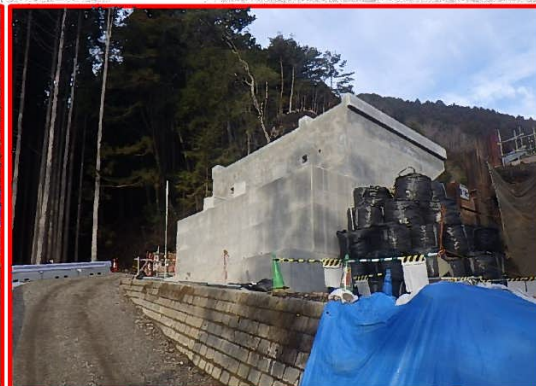
②橋梁下部工
