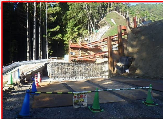
③橋梁下部工
