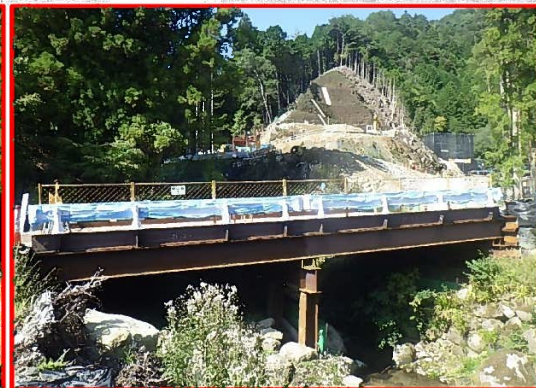
②橋梁下部工
