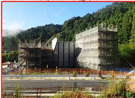
①大名倉区橋梁下部工
