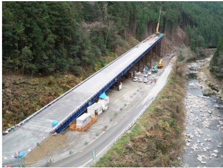
②廃棄岩骨材運搬路
