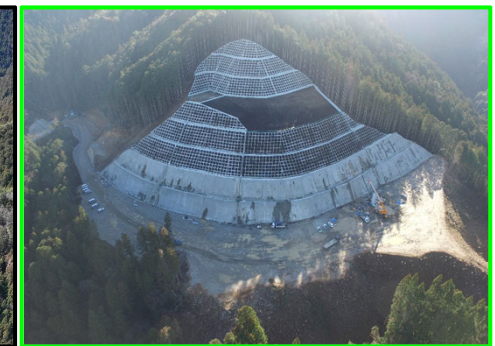
①左岸頂部掘削
