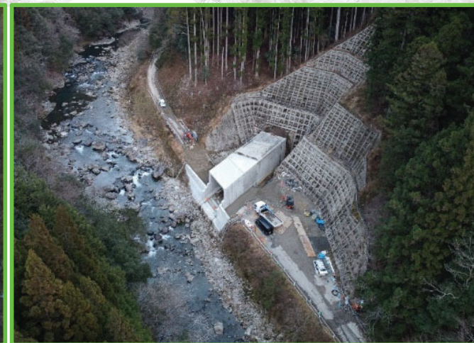
① 堤外仮排水路 (吐口側)
