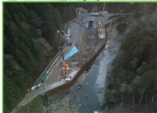
① 堤外仮排水路 (呑口側)
